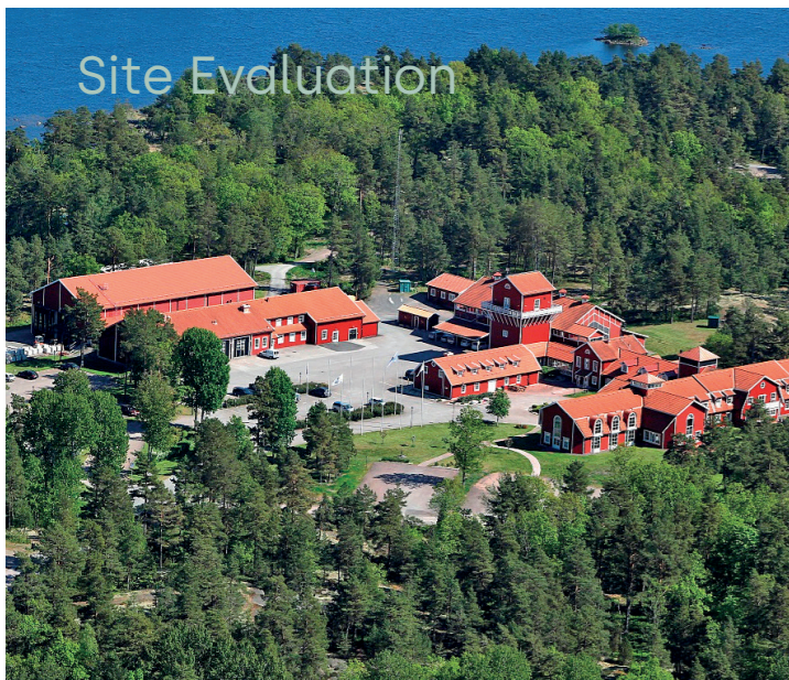
Surface facilities at Aspo Hard Rock Laboratory, Sweden (picture from SKB)
